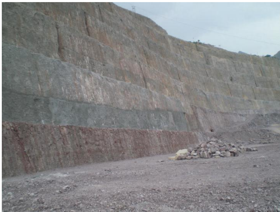
Figure 15 - Benches formed by Pre-split Blasting at Kol Dam Project
